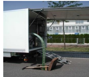
Inserting cable trays into sewers
