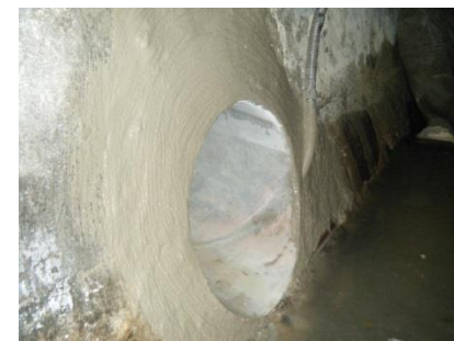
Establishing connections between sewers and buildings
