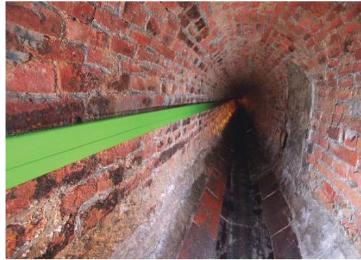
Modern network connections in old sewers
