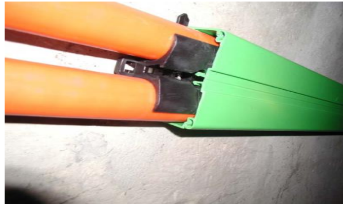
Easy installation process: Clips that are mounted on the wall carry the cables, a flexible cover offers additional protection
