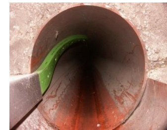
Robotic installation of cable trays in non-accessible sewers
