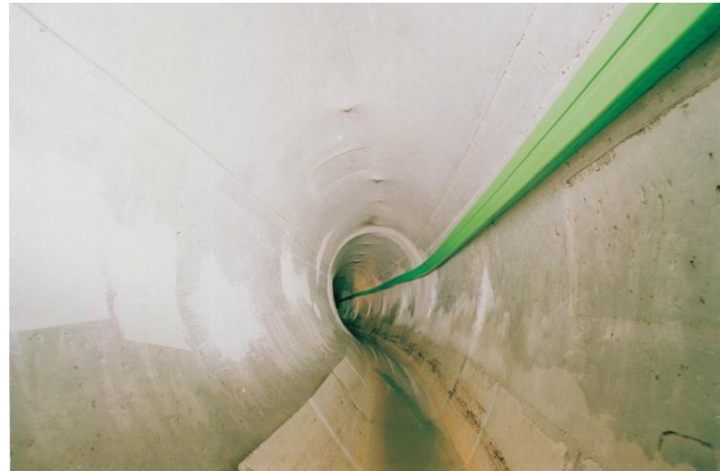
Vienna's backbone, installed with CableRunner technology
